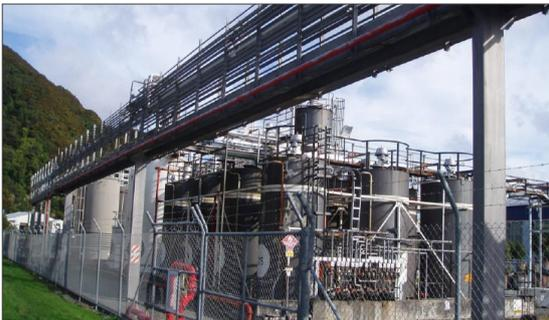
It is essential that certifiers of stationary container systems pay specific attention to the vents. This includes those certifiers who are approved for installation of tanks – it is **not** sufficient to assume that vent sizes were verified in the design of the tank as they may not have been.
