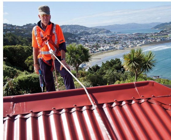
Figure 3: A safety harness and safety line used as a work positioning system
