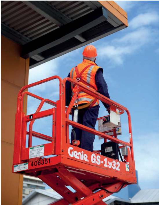
Figure 2: Powered access for inspecting a large fragile roof
