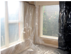
Create an enclosure before removing a textured ceiling containing asbestos.
