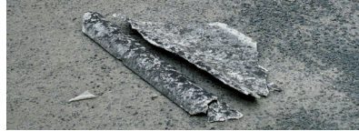
Non-friable asbestos may become friable after being damaged
